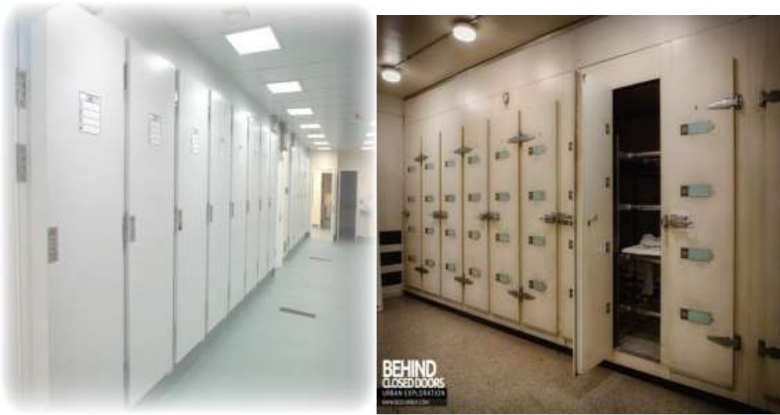
Fig 4: refrigerated body storage cabinet.
